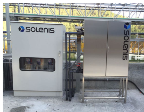
Dosing pump cabinet (left) and OnGuard™ 3S analyzer and OnGuard™ P controller (right)
