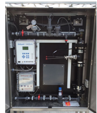
Dosing pump cabinet (left) and OnGuard™ 3S analyzer and OnGuard™ P controller (right)
