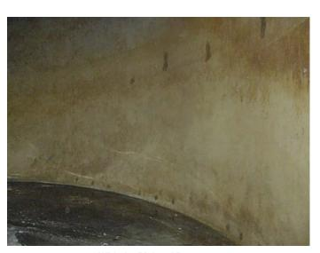
With the Biobond Program: whitewater chest walls clean, no deposition
