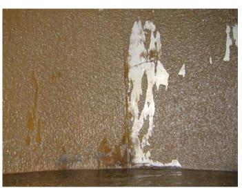
Without the Biobond Program: walls of whitewater chest show high levels of deposition
